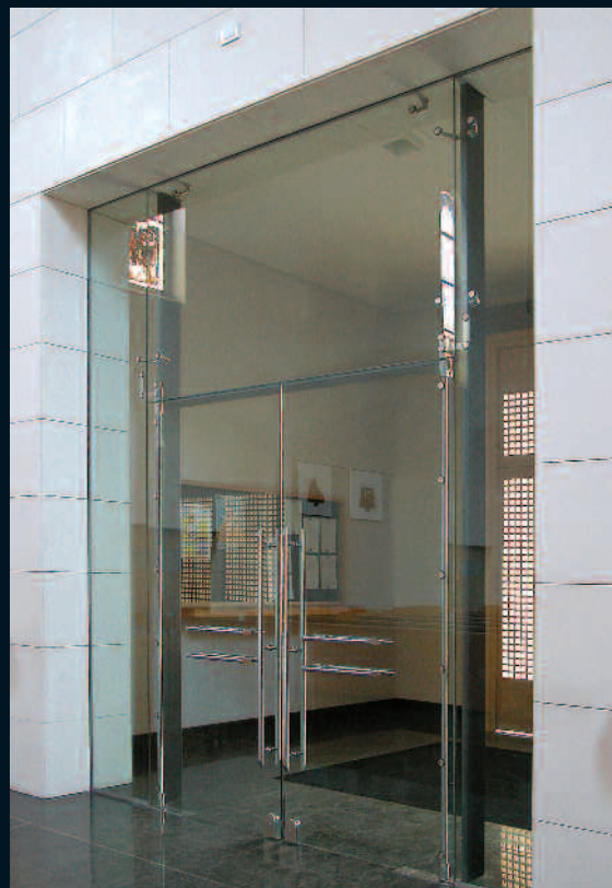
Entrance area of Don-Bosco Church, Bolzano, Italy (with cross formed by MANET pull handles)
